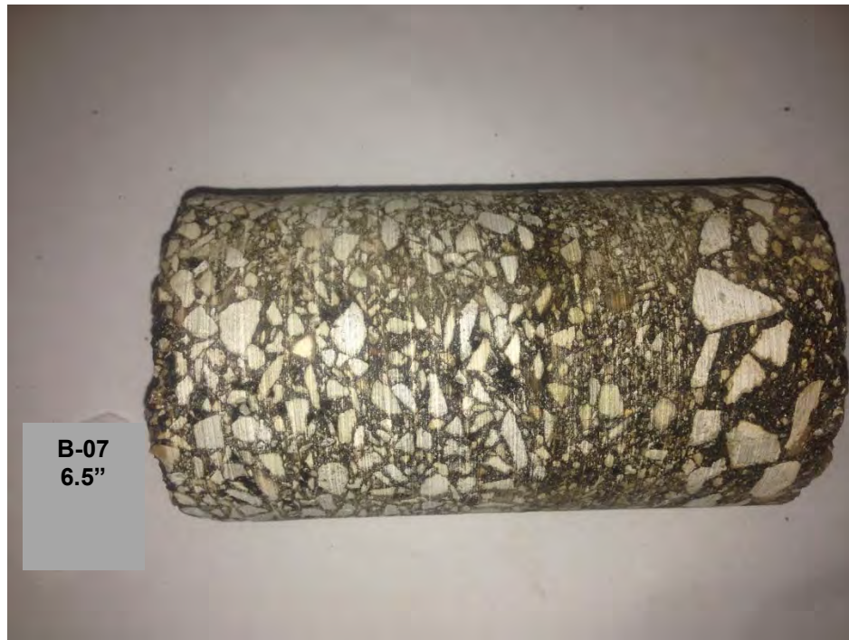
PHOTOGRAPH 21: Pavement core from B-07.
