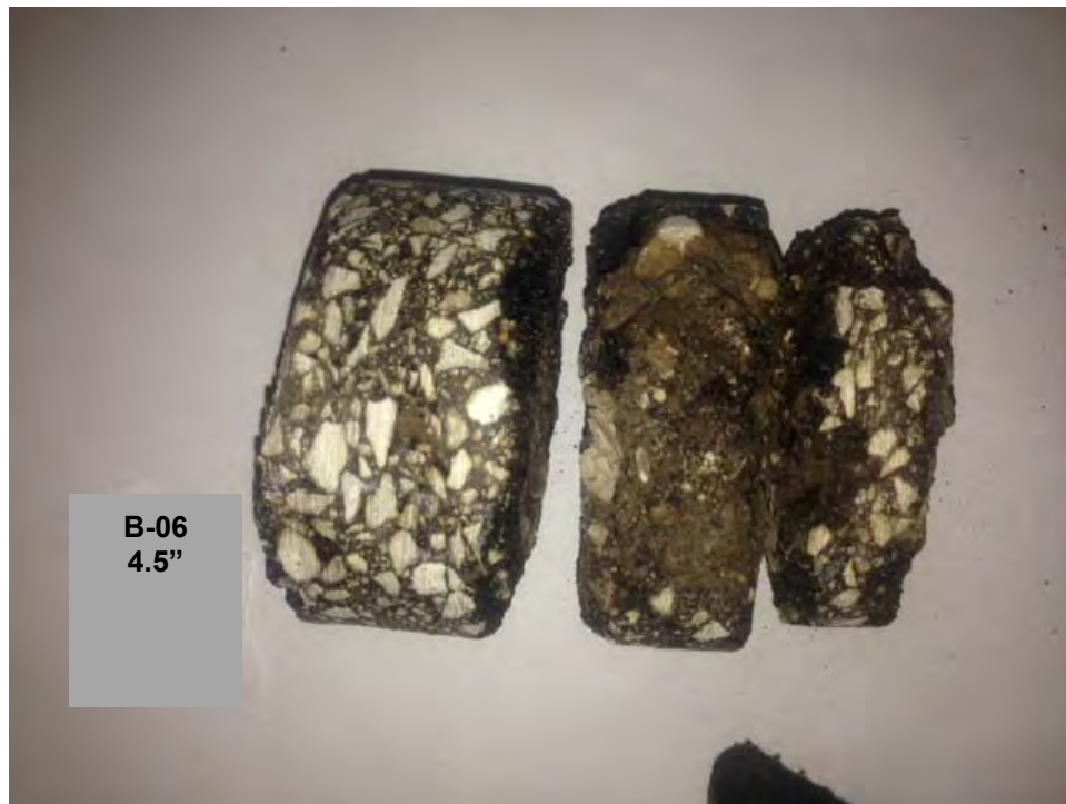
PHOTOGRAPH 20: Pavement core from B-06.
