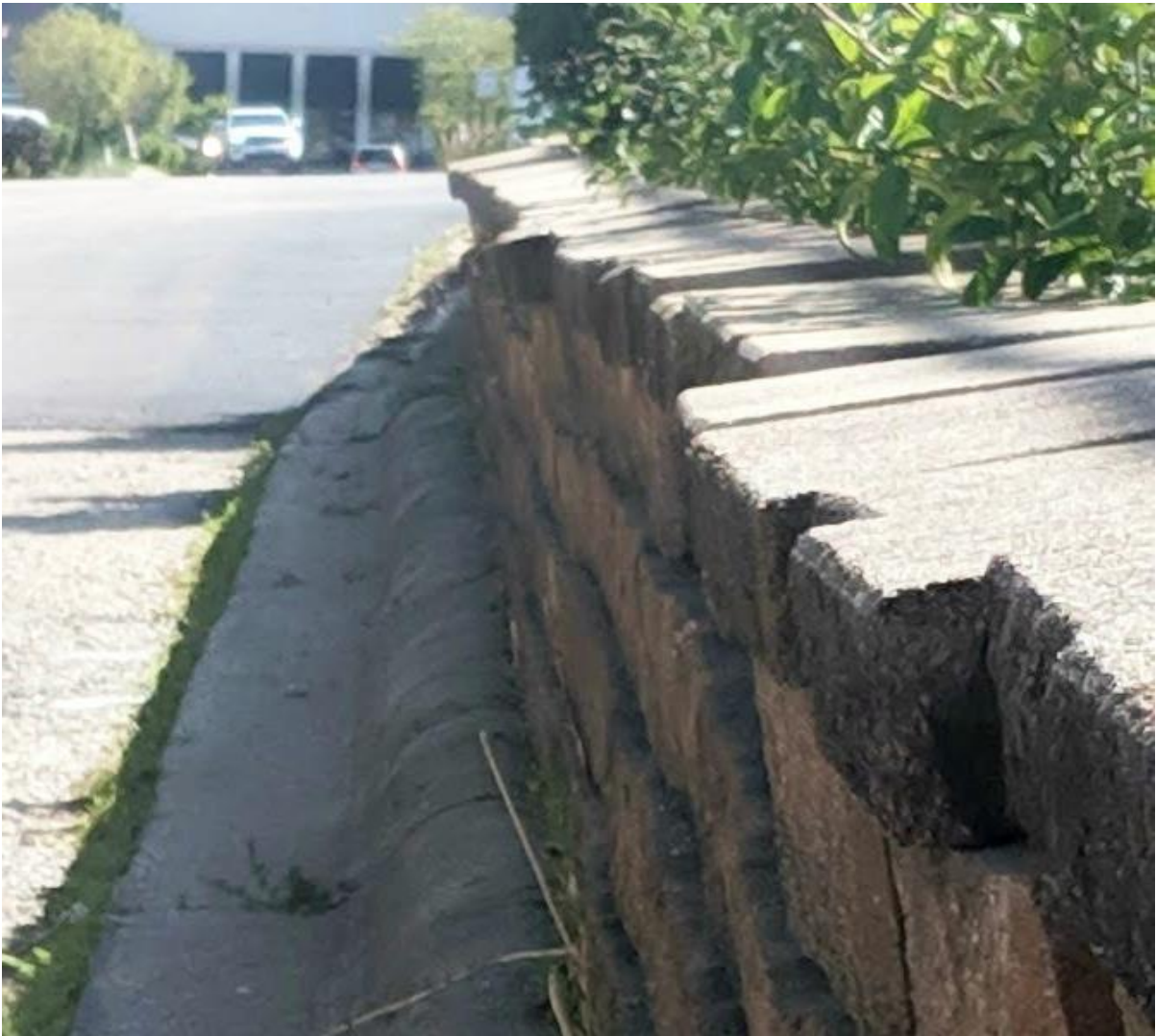
PHOTO OF RETAINING WALL LOOKING EAST
