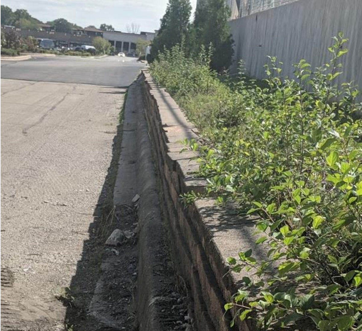
WIDER VIEW OF RETAINING WALL AT VILLA OAKS
