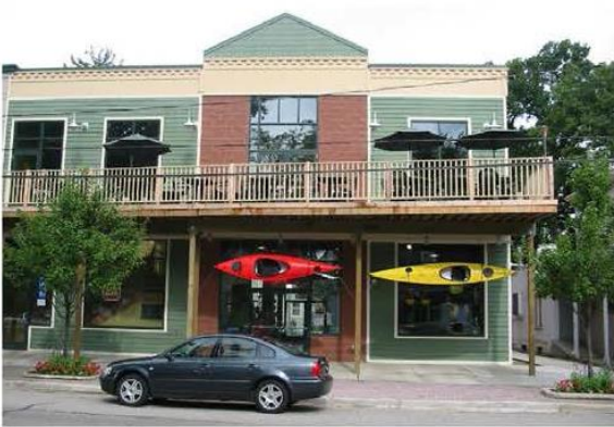
Primary Materials: Painted Wood
