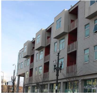
Figure 4-30 Balconies Integrate to Facade
