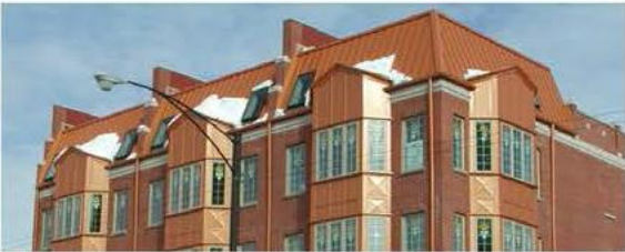
Roof Materials: Metal
