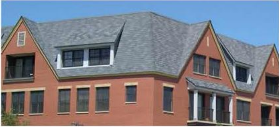
Roof Materials: Asphalt Composite Shingles
