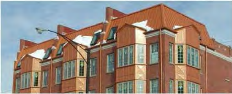
Roof Materials: Metal
