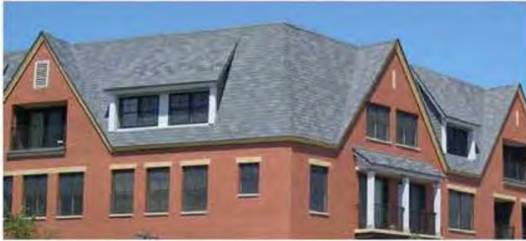
Roof Materials: Asphalt Composite Shingles
