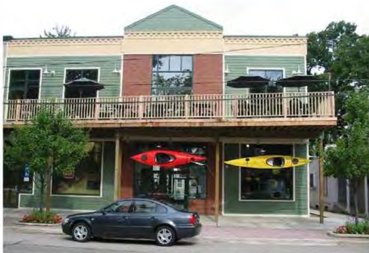
Primary Materials: Painted Wood
