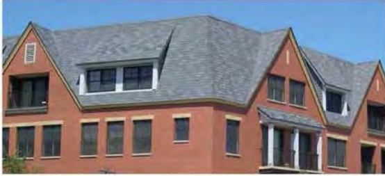
Roof Materials: Asphalt Composite Shingles
