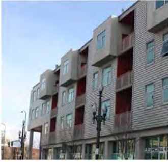
Figure 4-30 Balconies Integrate to Facade
