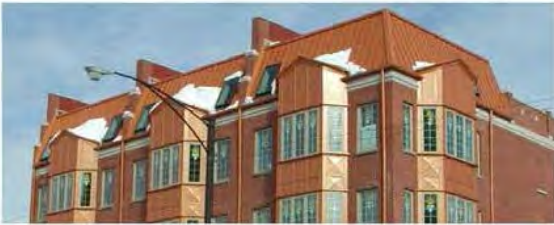
Roof Materials: Metal
