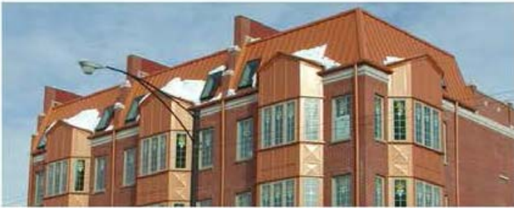
Roof Materials: Metal
