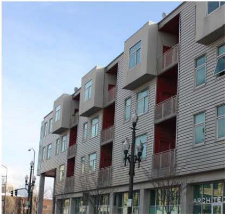
Figure 4-30 Balconies Integrate to Facade
