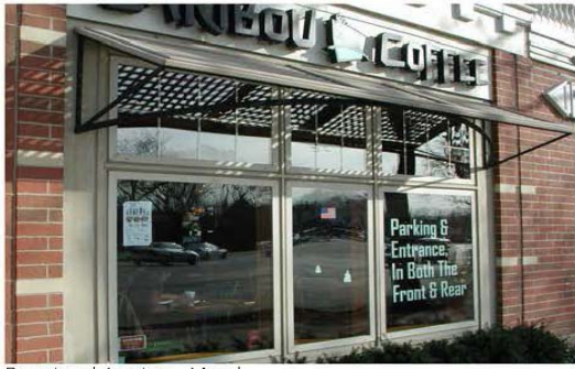
Permitted Awnings: Metal
