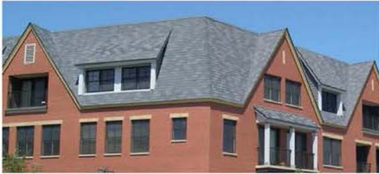
Roof Materials: Asphalt Composite Shingles
