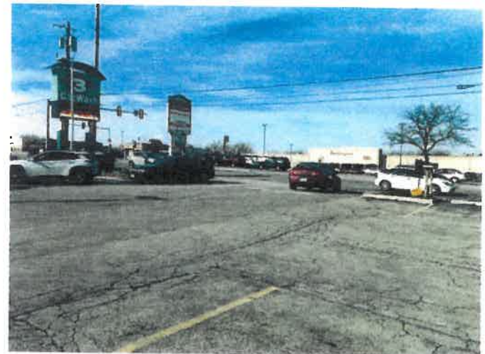
Looking north on Site Access driveway, south of IL 38
