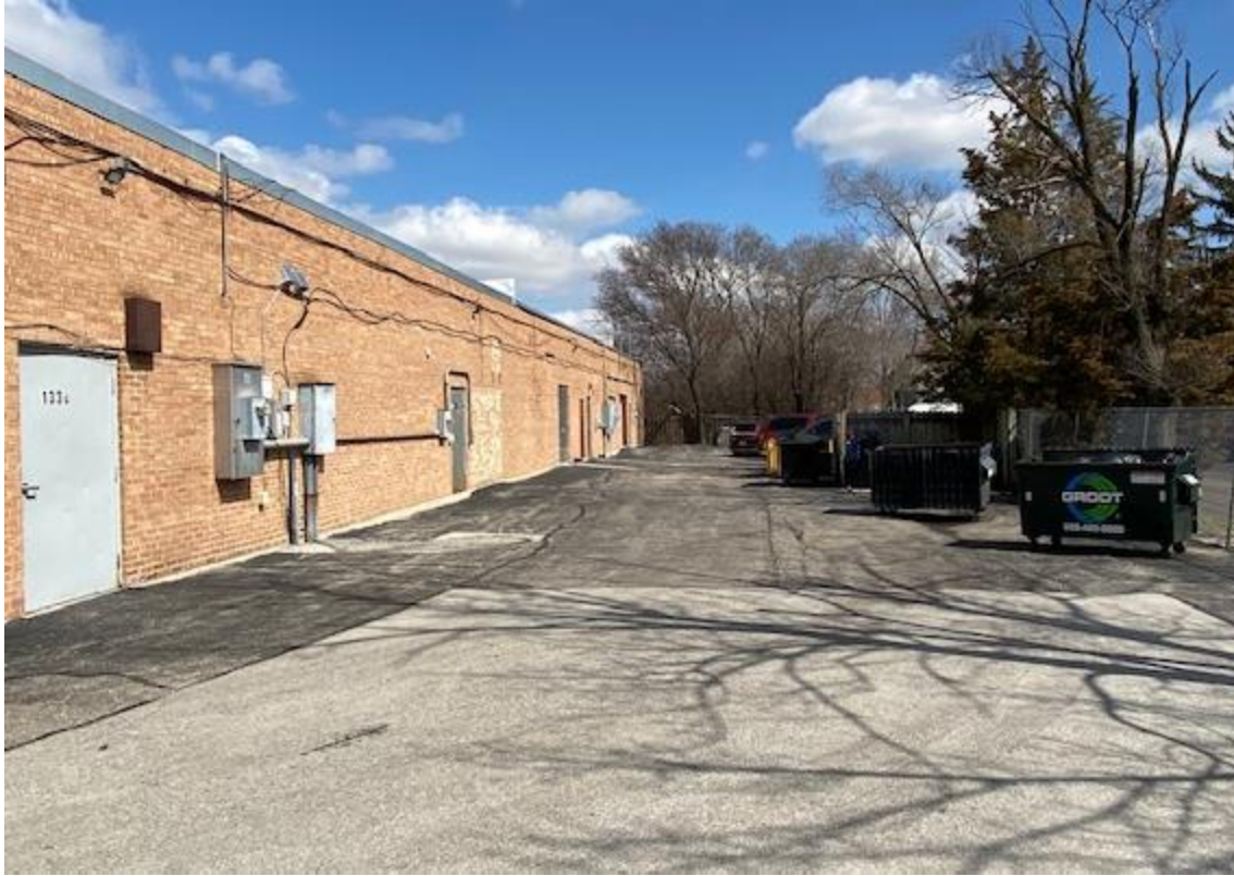
REAR OF THE SUBJECT SITE (SOUTH SIDE)
