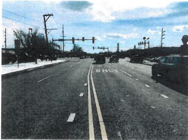
Looking south on Ardmore Ave, north of IL 38
